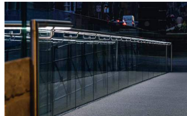
Example of concealed lighting with handrail
