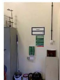
Level 04: Stair B Lobby
