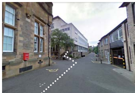
2. Main Entrance to Kelvin Building
