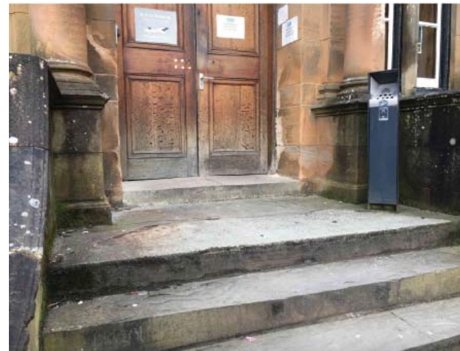
2. Main Entrance Door 2 - Entrance at South Facing Elevation (non accessible entrance)
