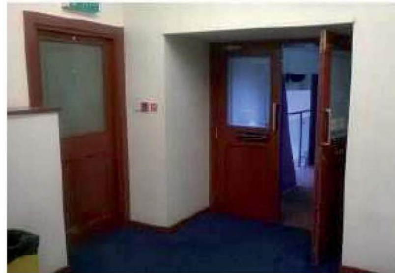
Existing entrance into common room (level 4)
