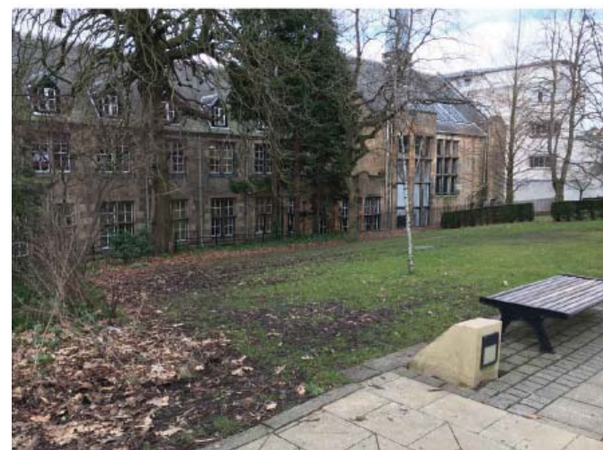
6. The Kelvin Building East Facing Elevation / landscape strip
