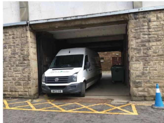
5. Courtyard/ Deliveries/ Access below pend/ accessible entrance (Entrance Door 4)
